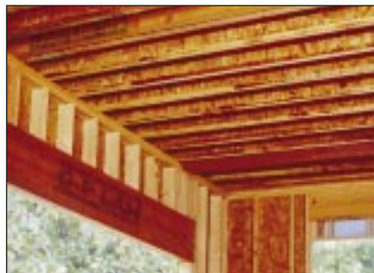
Wood I Beam joists help eliminate the need for support posts in basements, garages and bonus rooms.
