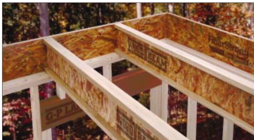
Wood I Beam joists help eliminate the need for support posts in basements, garages and bonus rooms.
