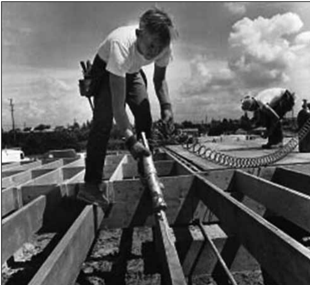
Figure 10–7. A pressurized extruder applies a single bead of elastomeric construction adhesive to floor joists for assembly of a plywood floor system.
