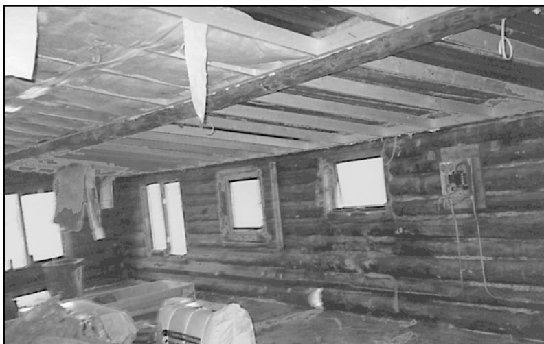
An interior retrofit of a ceiling in progress; note new electrical wires being installed.
