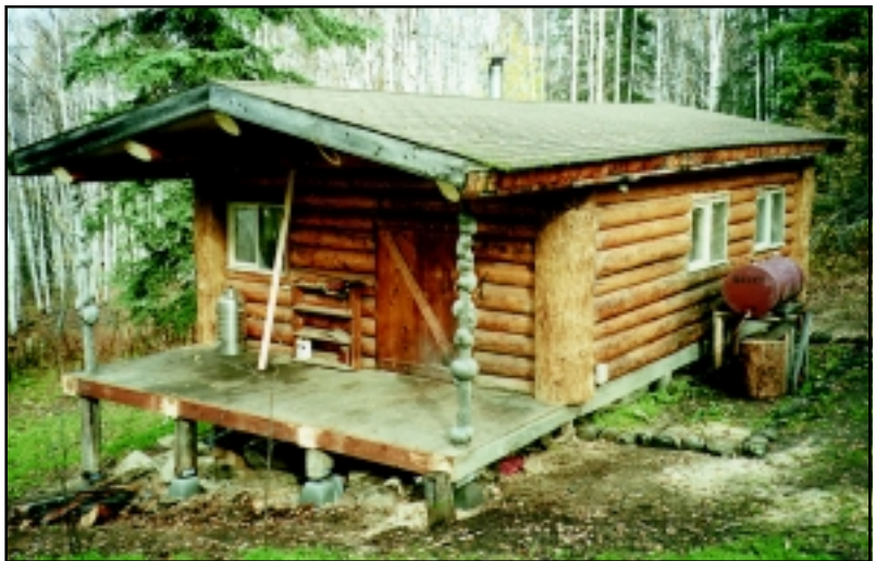
The cabin was saved by cutting out all four log corners and installing large vertical log corner posts. A good solution to use as much of the old building as possible. Note the trimmed roof logs and shorter porch.
