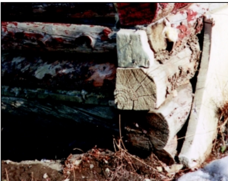
The lower logs of buildings in ground contact will often be rotten beyond use and must be replaced.
