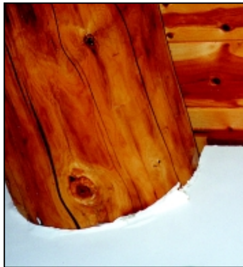
This ridge pole, which rests on a horizontal log gable, shrank and settled more than 6 inches and is now crushing the Sheetrock.
