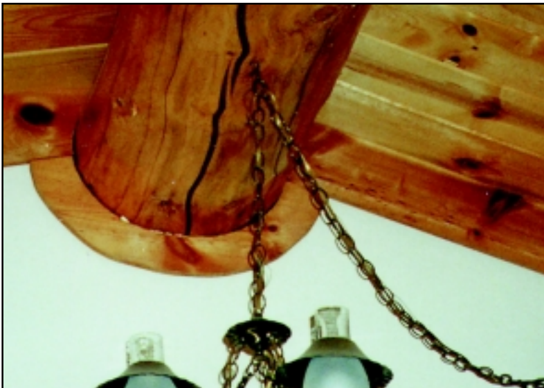
The gap left for settling here is covered with scribe-fit trim.
