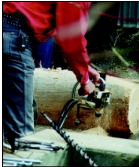
No exhaust fumes is one benefit from using hydraulic chain saws indoors during winter construction.
