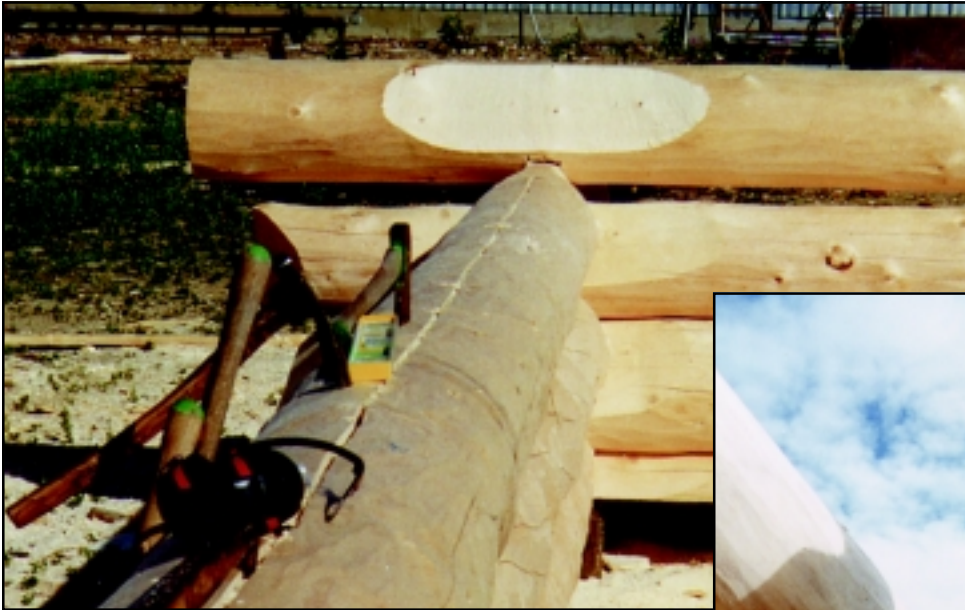
Scarf is sanded smooth, ready for final scribing. Note stress relief kerf on top of logs to promote controlled checking.
