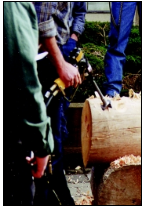
A hydraulic drill being demonstrated at a log building conference. Note the one-handed operation.
