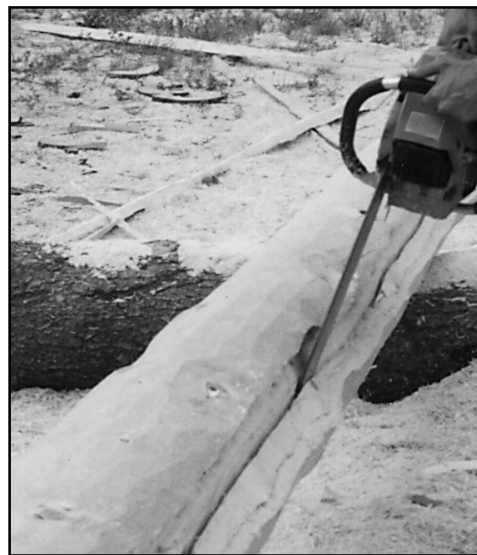
Cutting the groove with a chainsaw.
