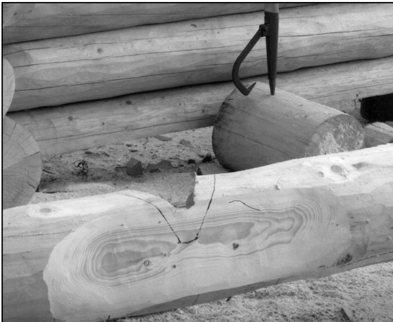
The final scribe is visible on this log on the skids, ready for cutting.
