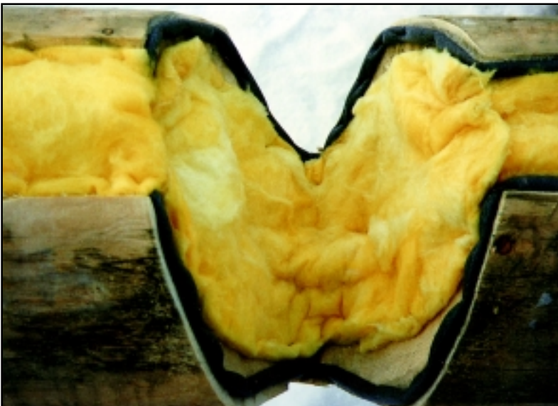
Both fiberglass and backer rod installed on a log.
