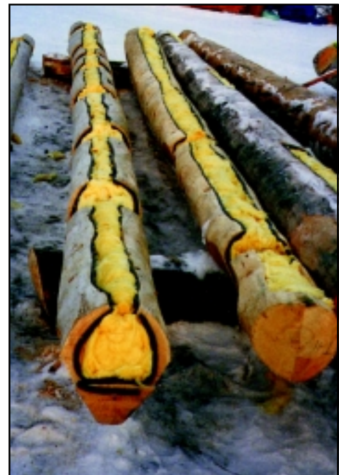
Logs ready to be lifted into place.
