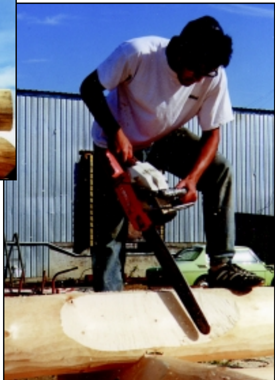
brushing with the chainsaw to smooth the scarf
