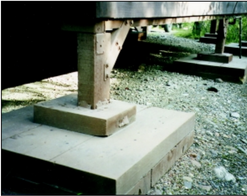
A nice-looking post and pad foundation installed near Fairbanks.
