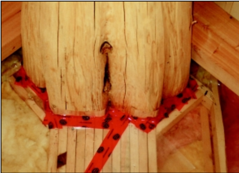
Sealing the vapor barrier around a log ridge pole.
